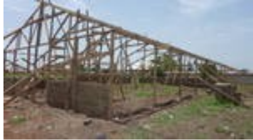
Open Door Church being built in March 2010 in Nsoatre, Ghana.
