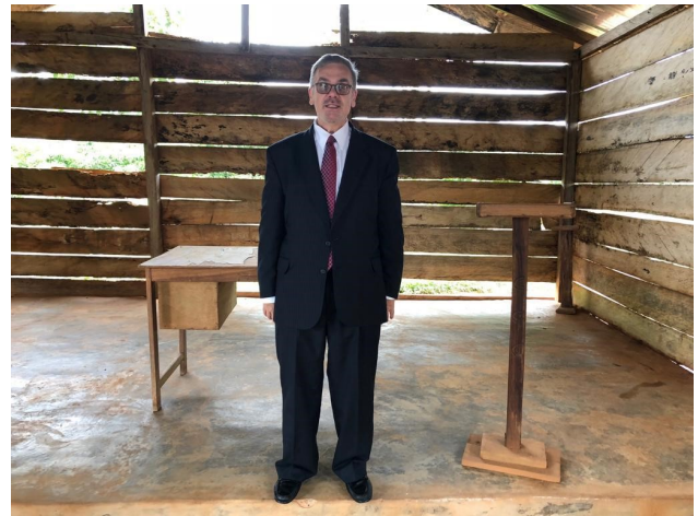
This was taken inside the building last October. Notice the poor condition of the wood and the walls. Only the front had concrete, the rest of the floor was dirt.
